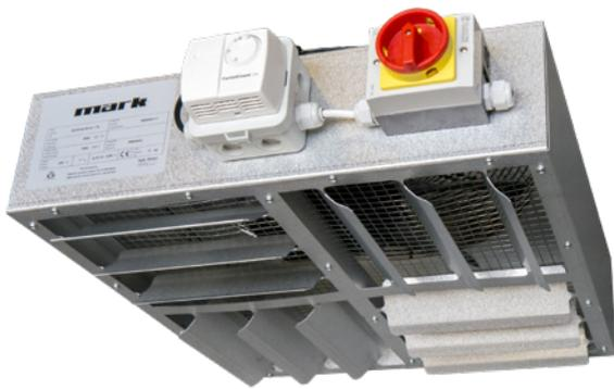
Mark recommends an ECOFAN with every air heater. A combination of these products provides optimum comfort and good heat distribution within the room. It is known that hot air rises which means that an air heater requires more time to heat up a room. A thermostatically-controlled ECOFAN transports the warm blanket under the roof to the occupied area. As a result, the room heats up more quickly, and gas consumption can in some cases be reduced by up to 30%.
